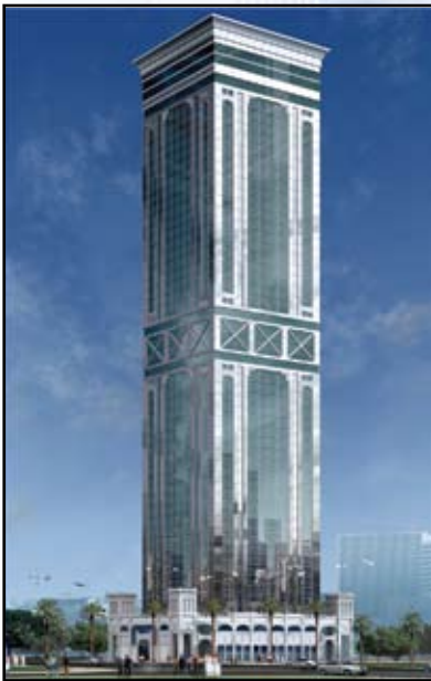
AI Fardan Residence, 3B+G+61+R Location Doha, Qatar
