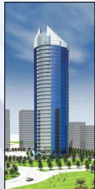
Yohan Tower (2B+G+32+R+UR) Location Doha, Qatar
